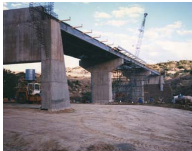
FAR LEFT: Composite bridge, Nigeria. One of several multi-span complete bridges supplied by us on the Wawa-Kaima road.
