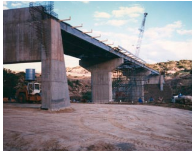
Far Left: Composite bridge, preparing to launch in Uganda.
