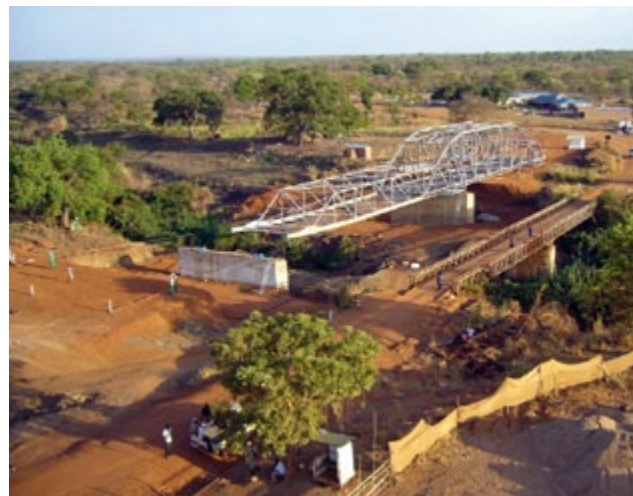
Far Left: One of our 50 metre clearspan, two lane roadway bridges on the Aweil Road, Southern Sudan.
